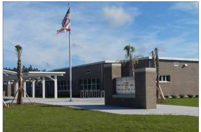
Photo of Wildlight Elementary School.
